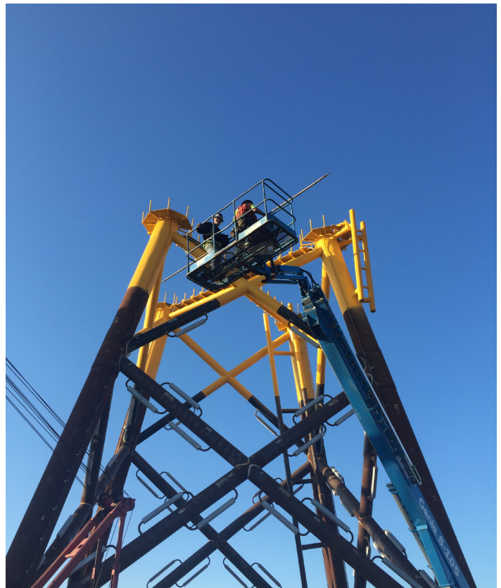
Photo credit: Dan Clark, Pile Drivers Local 56/Weeks Manson
